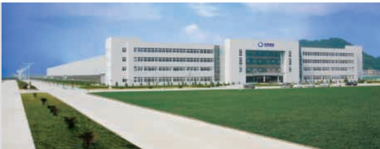
新落成的路橋廠房 Newly completed Luqiao plant
